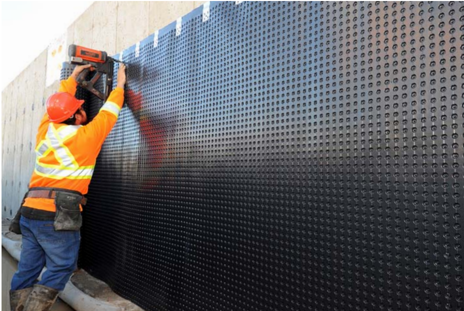
INSTALLING SPEEDCLIPS EVERY 30CM (12")
